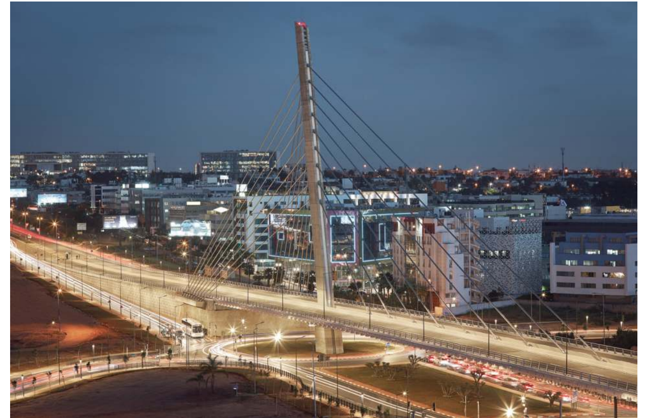
↙ Casablanca Sidi Maârouf cable bridge
